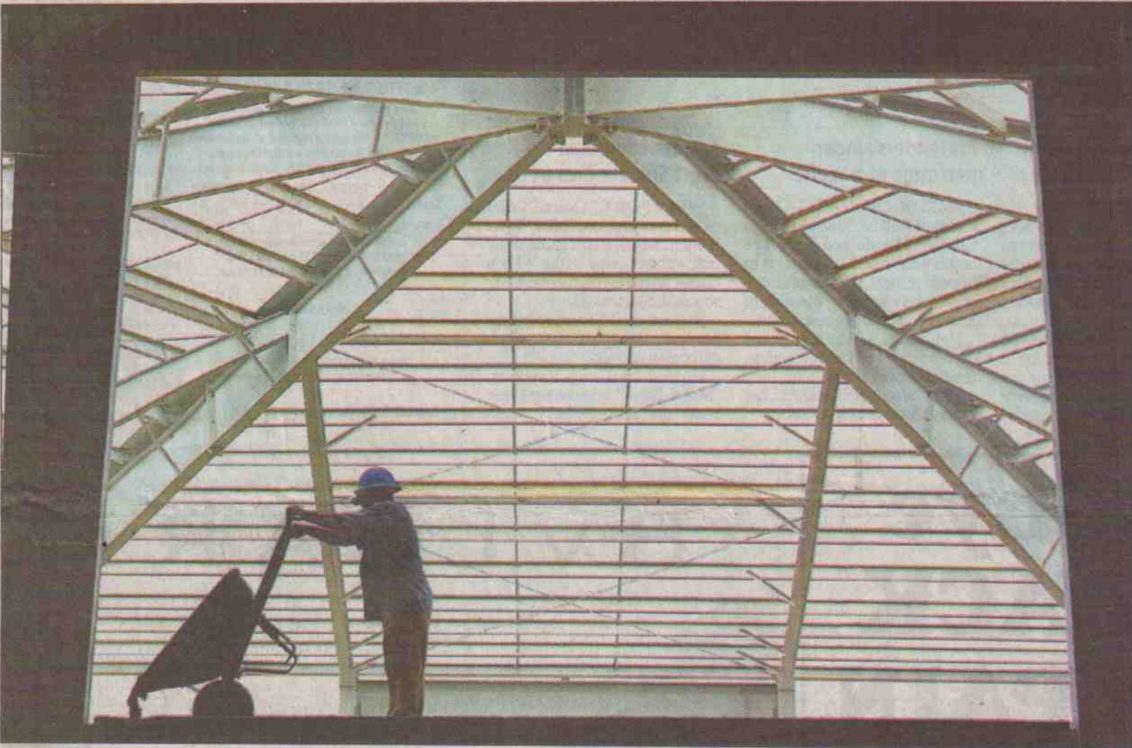
Tradesman Joe Soliz spreads mortar on the second floor of the food arena at the Naples Big Cypress Market Place on Sept. 7. The 87,000-square-foot shopping and entertainment center on U.S. 41 East in East Naples is scheduled to open in November. David Albers/Staff (2)
