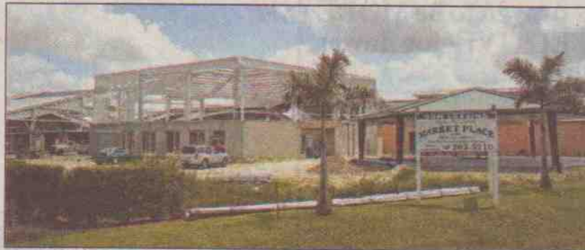
Construction continues at the Naples Big Cypress Market Place. A little smaller than a Wal-Mart, the shopping and entertainment center will include an indoor flea market, winery, entertainment area and convention center.
